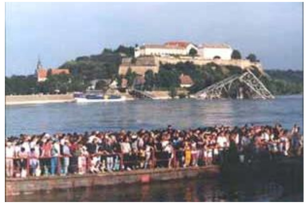
Fig. 4 Varadin Bridge on April 15 th , 1999
